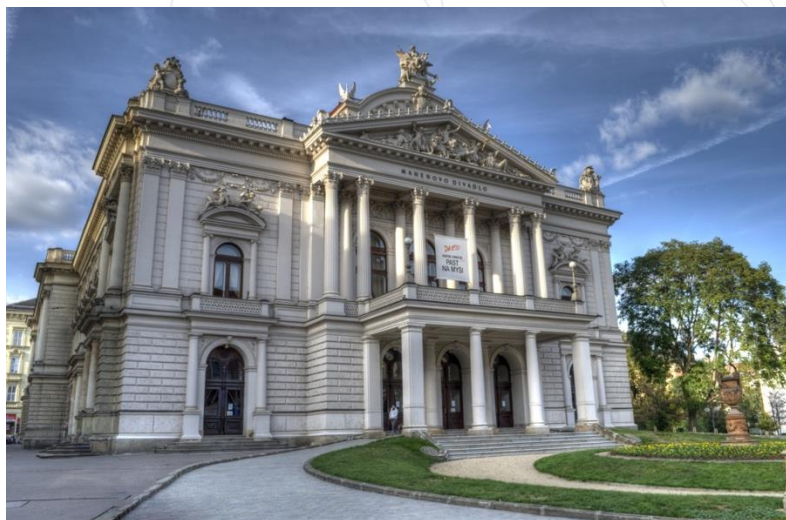
National Theatre Brno Mahen Theatre
